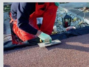
\* Please note that the calculation of the weight for the grit/gravel is only an approximation. The materials used are natural building materials and are therefore subject to natural fluctuations. When compacted, the volume decreases, by what the demand/quantity increases. Note on the surface depth: The surface should be three times as deep as the largest grain of the grit/gravel used to obtain a homogeneous and stable surface.
