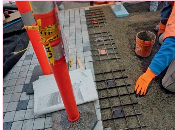
Precise laying of stones
