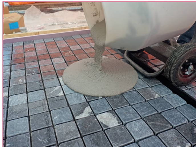
Working in the grouting compound
