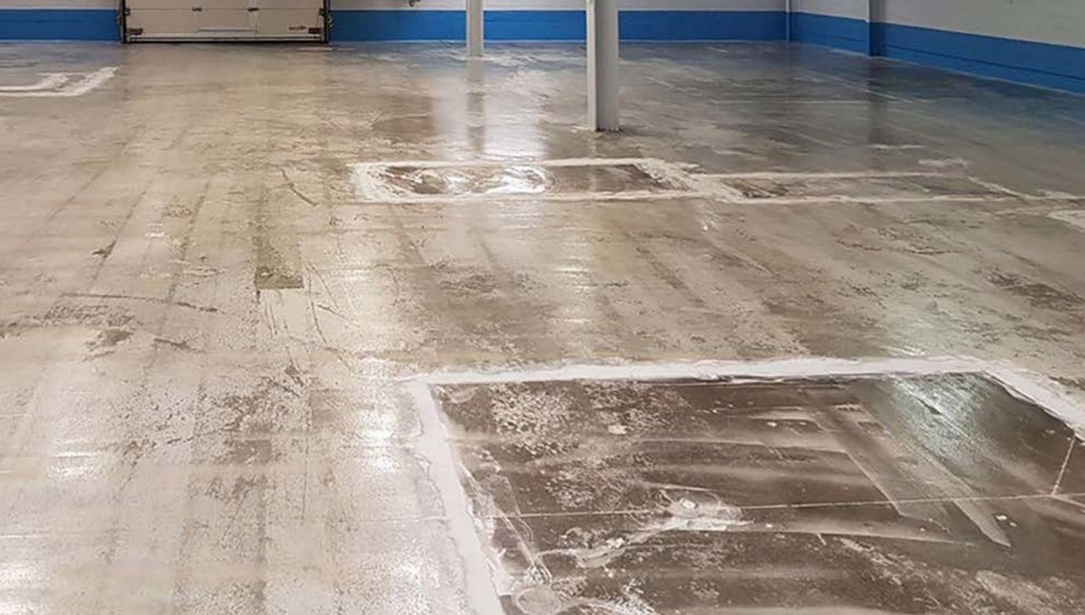
Surface before coating
