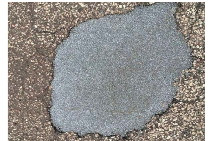
Filling of holes and damage
