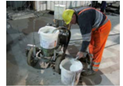
Example of a piston airless machine being used
