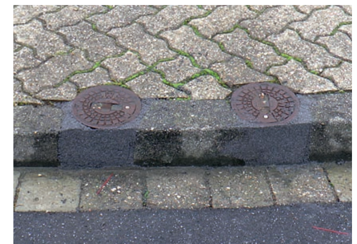
Repair of curbstones
