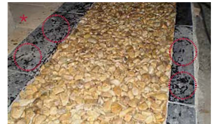
Synthetic resin marks on surrounds
