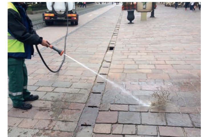
Cleaning of joints
