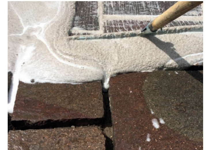
Repairing old cement joints
