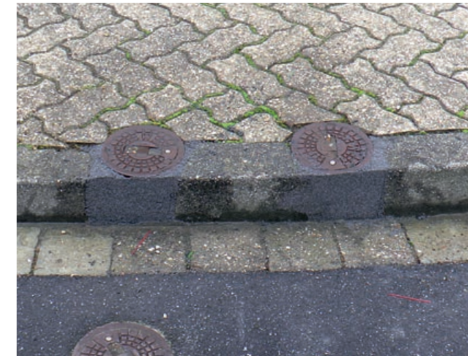
Asphalt repair and curbstone repair
