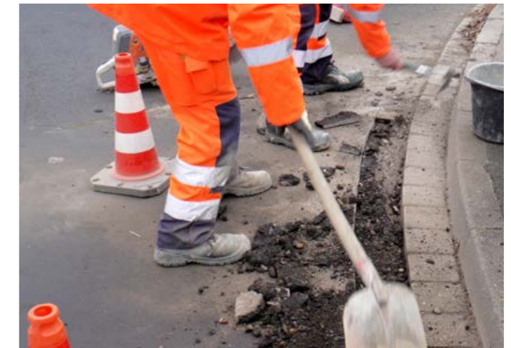
Repair of road damage
