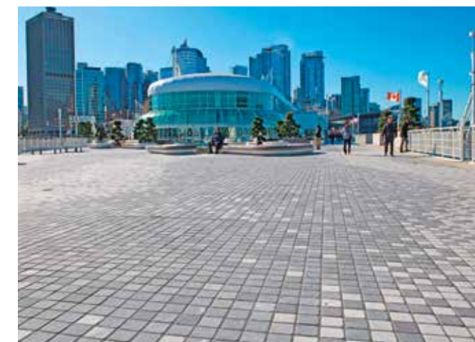
ROMPOX® - D1 installed on a natural stone commercial plaza
