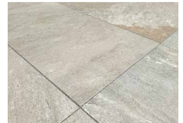
ROMPOX® - ECOFINE installed on porcelain tile residential patio
