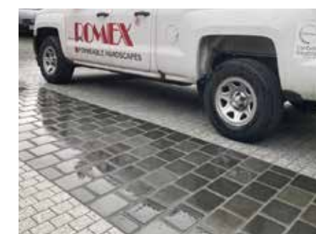
ROMPOX® - D1 installed on natural stone residential driveway
