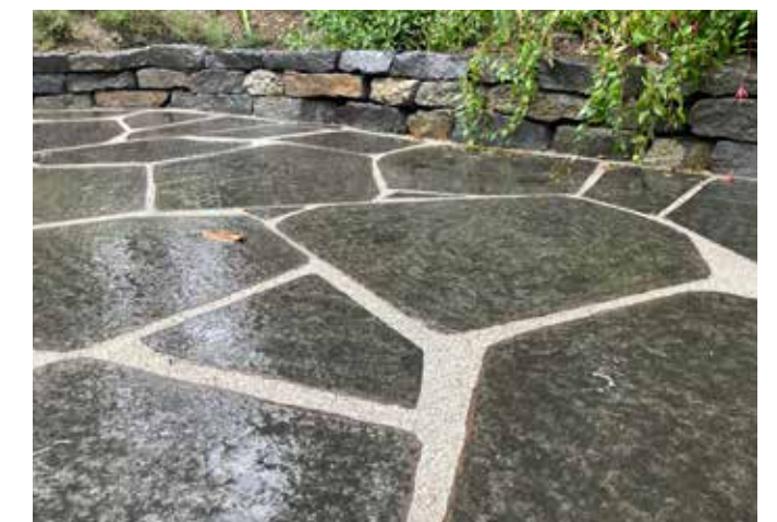
ROMPOX® - EASY installed on natural stone residential patio
